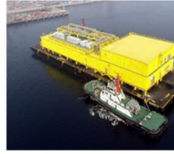
UZ750 Island Surface Facilities Modular Building Fabrication
