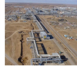
KOC Lower FARS Heavy Oil Packaged Substation
