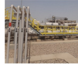
42" Onshore Export Pipeline at West Qurna Field
