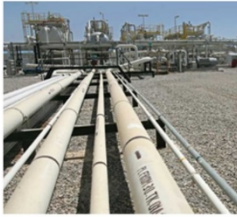
KOC Effluent Water Injection Project
