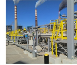
EPC for Badra-Zubaida Gas Export Pipeline Project
